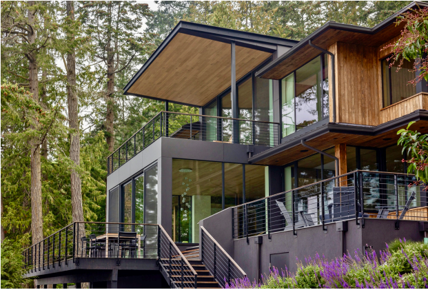
Custom steel handrails and details White Oak soffits at Entry & Upper Deck
